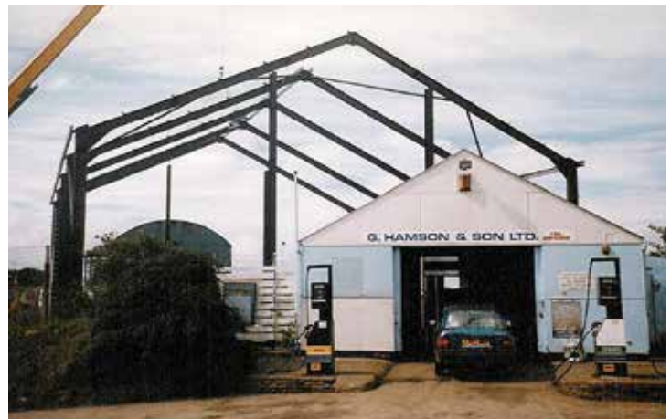
The new garage being built
