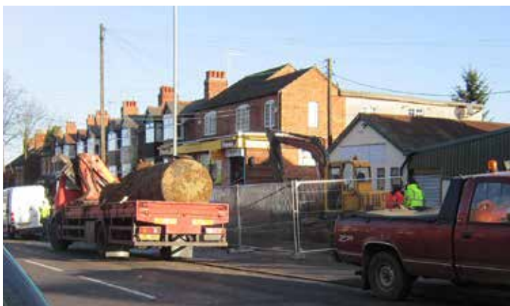
December 2011. The old petrol tanks are removed from the forecourt of the former premises in Northampton Road.
